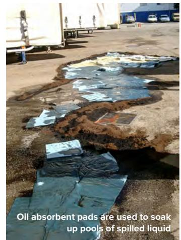
Oil absorbent pads are used to soak up pools of spilled liquid
