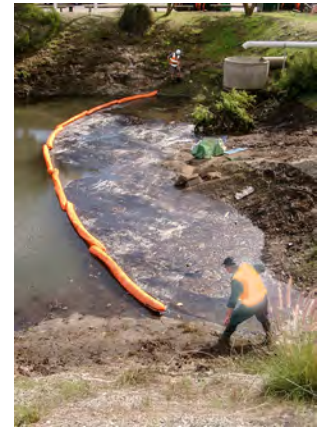
Booms contain the spill, absorbent peat encapsulates the spill.
