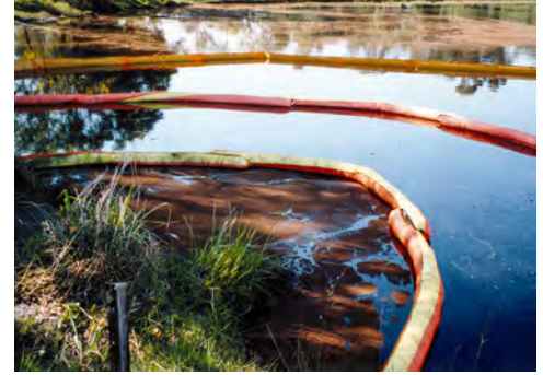
Booms contain the spill, absorbent peat encapsulates the spill.
